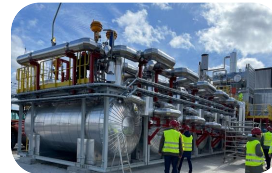
KYOTO™ 4 MW/18 MWh molten salt-based thermal storage system in operation (Denmark)
