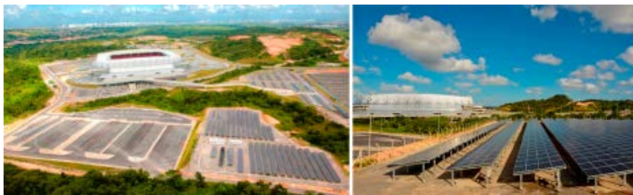
Solar Photovoltaic Power Plant
