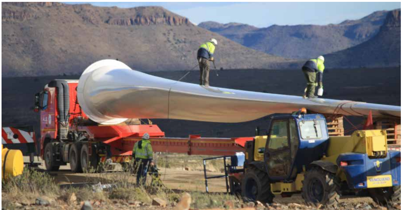
Wind turbine blade transport and anchoring work
