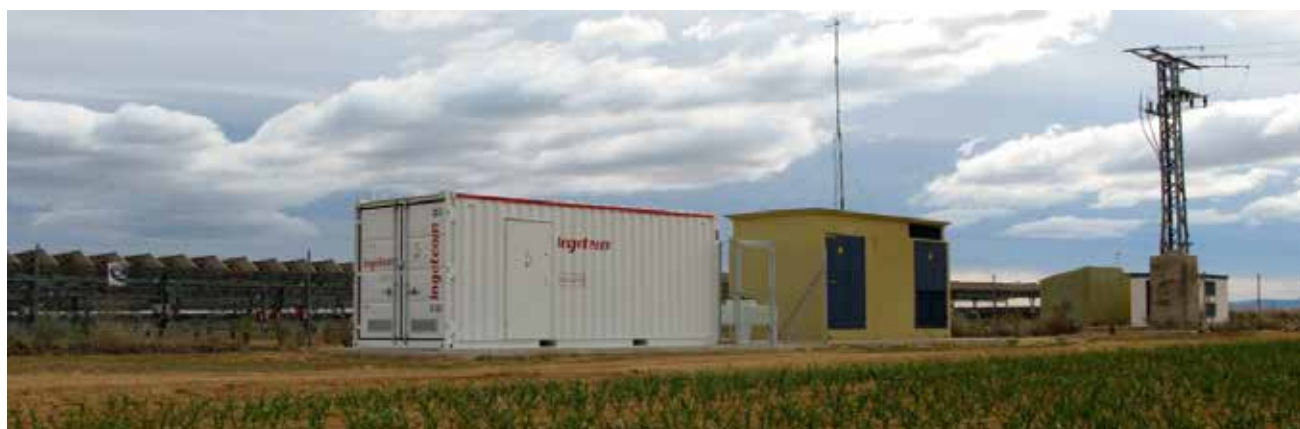
MV STATCOM (PV solar farm, La Herrera, Albacete)
