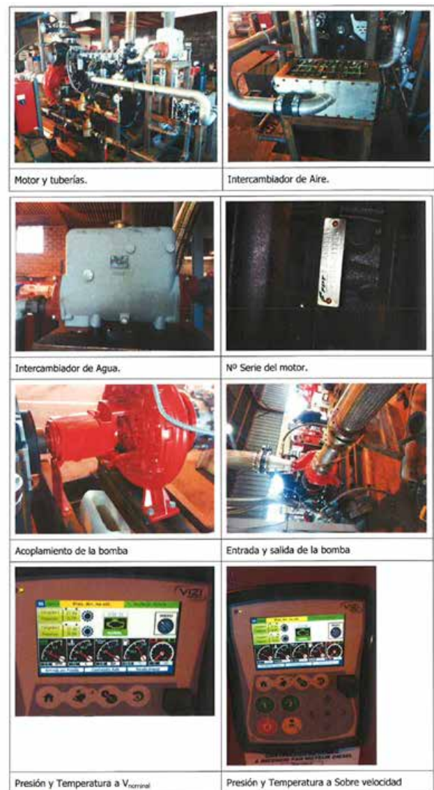
Elements constituting the pumping system and control panel
