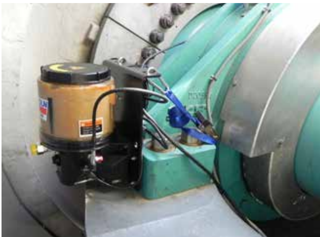
Rotor bearing self-lubricating system
