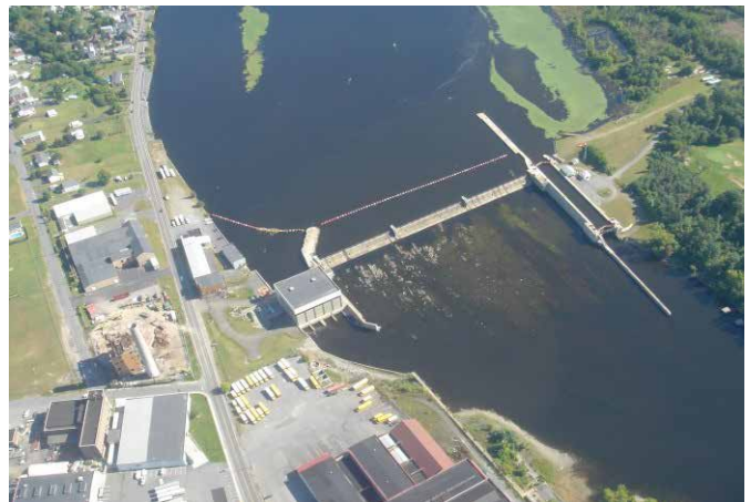
NYSEG Upper Mechanicville Hydroelectric Facility
