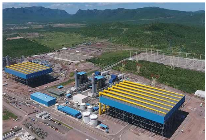
Noroeste 42 Topolobampo II Combined Cycle Plant
