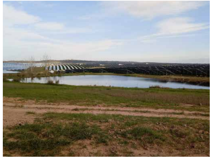
Pond inside the plant
