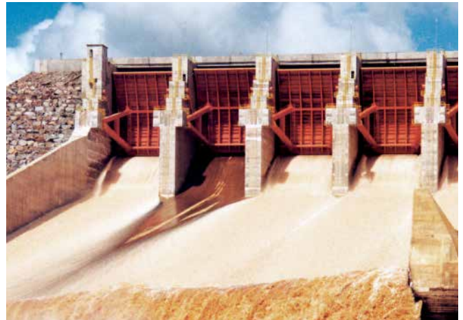
Itapebi Hydroelectric Power generation
