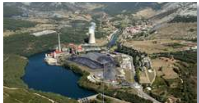
The Velilla Power Station
