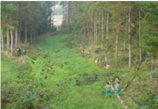
Vegetation management work
