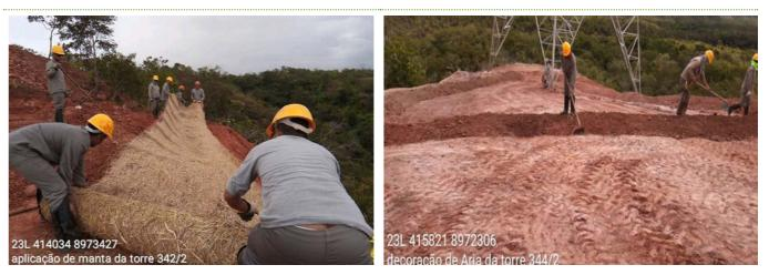
Application of sisal blanket as a containment measure - Tower 342/2 Installation of drainage devices as an erosion containment measure-Canteiro Monte Alegre do Piauí - 19/04/2021 Tower 344/2 Canteiro Monte Alegre do Piauí - 22/04/2021
