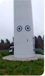
In 2020, a new surveillance system project based on artificial intelligence began. A 3D Radar is used with high resolution cameras that include an artificial intelligence system capable of detecting and identifying the position of the bird, its species and its trajectory. This allows the risk of collision to be analysed in real time, allowing the wind turbine to be stopped. In 2022 and 2023, work has been done on adjusting the system and verifying its effectiveness.
