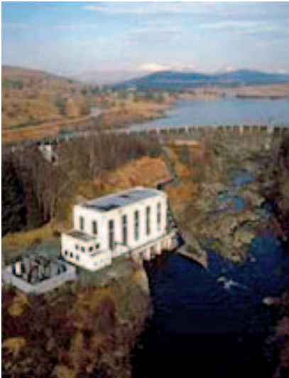
Galloway Hydro Power Station (Scotland).
