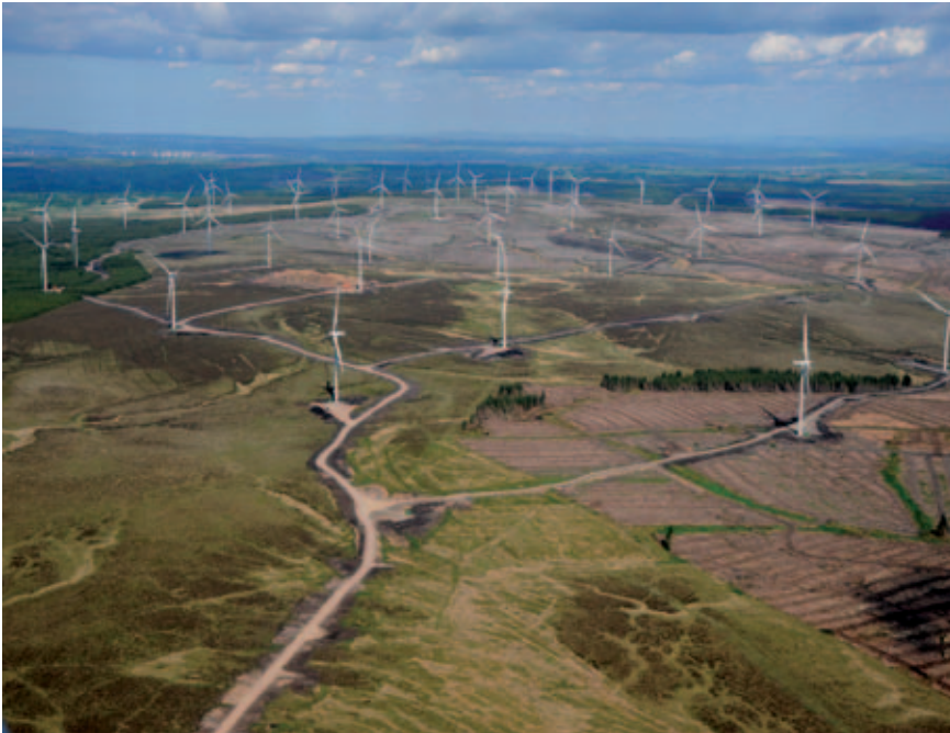
Whitelee Windfarm (Scotland).
