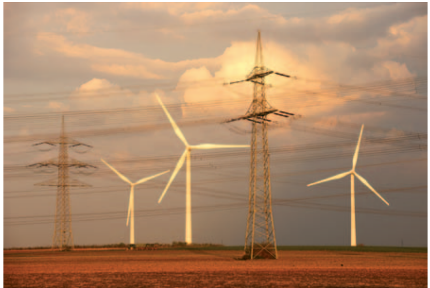
Windfarm and networks.
