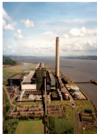
Longannet Power Station (Scotland).
