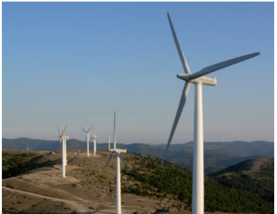
Thrace Windfarm (Greece).
