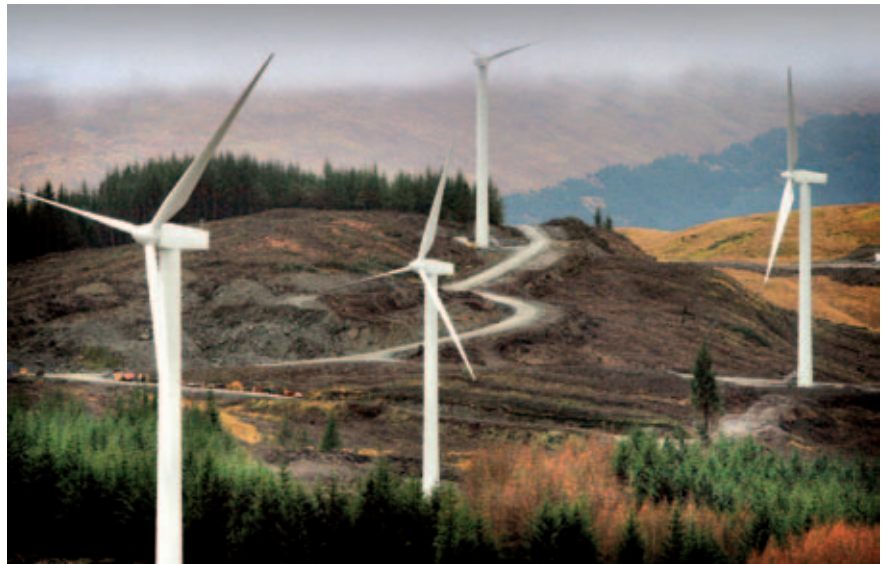
Cruach Mhor Windfarm (Scotland).
