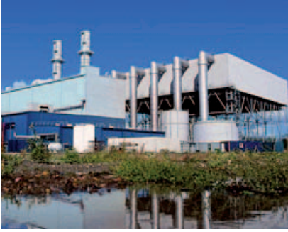
Damhead Creek Power Station (England).
