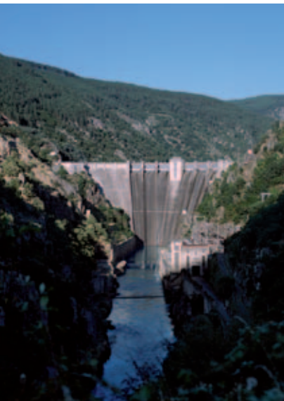
San Esteban Hydro Power Station (Orense).
