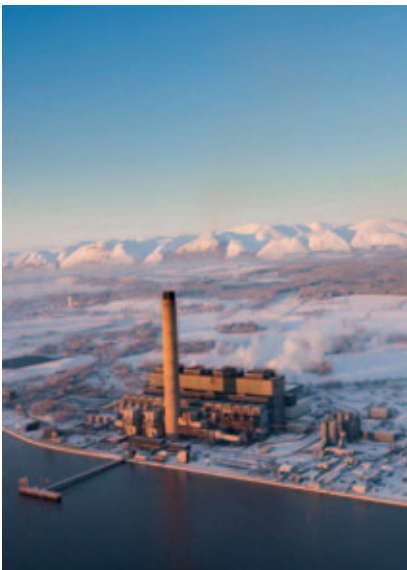
Longannet Power Station (Scotland).
