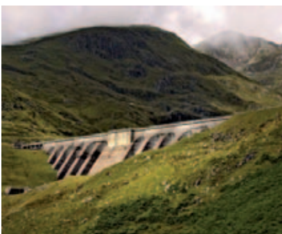
Cruachan Hydro Power Station (Scotland).
