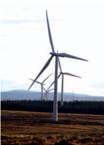
Whitelee Windfarm (Scotland).
