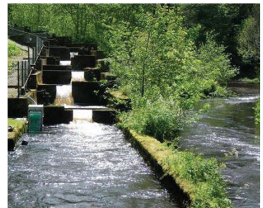
Figure 3: Trap 1 located beneath the fish pass
