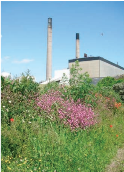
Cockenzie Thermal Plant
