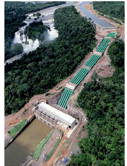
Dardanelos Hydroelectric Plant (Brazil).
