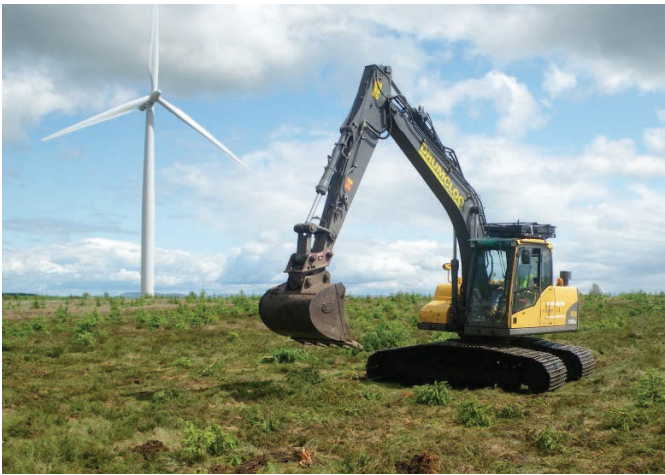
Excavator flattening plough/furrow features on drying bog surface and visible standing water 6 months later.
