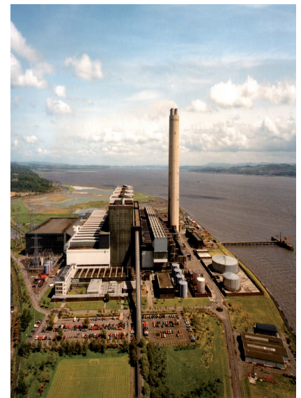
Longannet Power Plant (Scotland).
