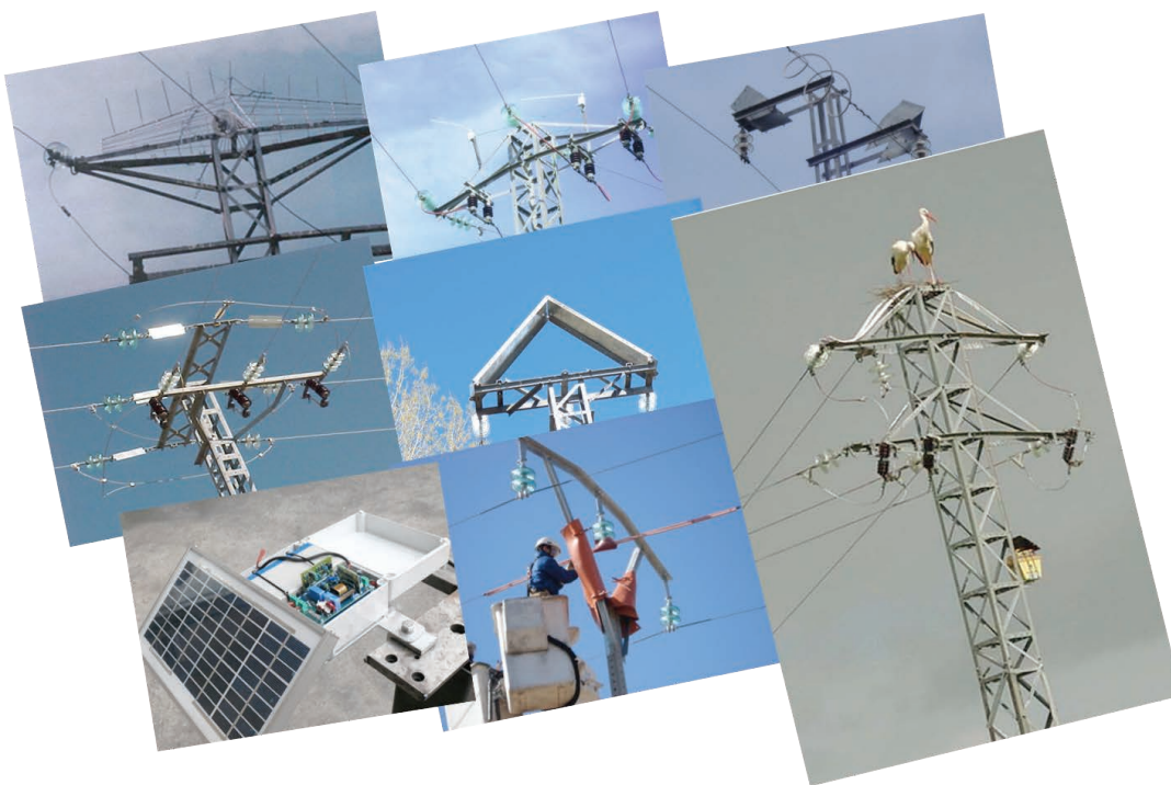
Protective elements installed for birdlife
