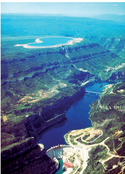
Cortes Hydroelectric Plant - La Muela I and II (Valencia)
