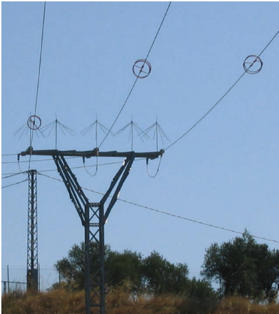
Power line umbrella anti-perching and anti-collision deterrent devices.
