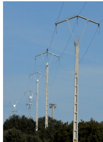
Power line with Wigeva crossheads preventing birds from perching and nesting.
