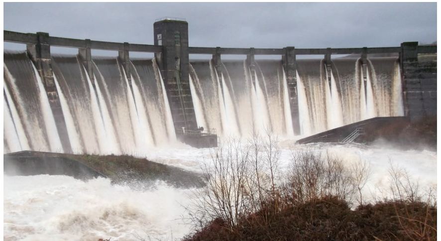
Opening the Carsfad reservoir gates at the Galloway hydroelectric complex (UK)
