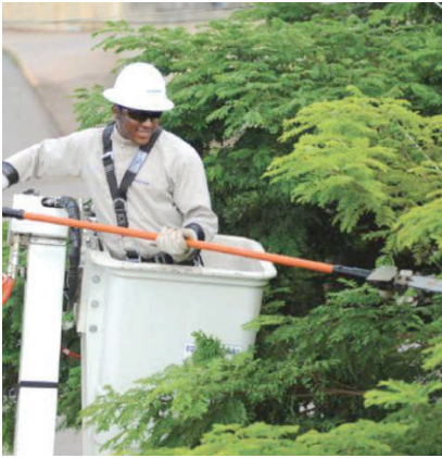
Power line tree trimming
