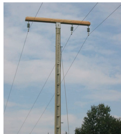
Model patented by IBERDROLA for reducing the risk of bird electrocution.
