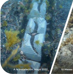
Protection of submarine cables with concrete blocks with ecological design
