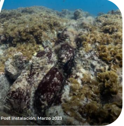
Protection of submarine cables with concrete blocks with ecological design
