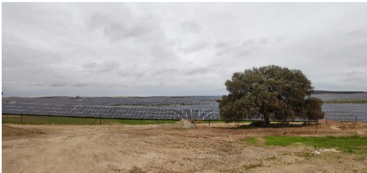
Francisco Pizarro photovoltaic power plant - Cáceres, Spain
